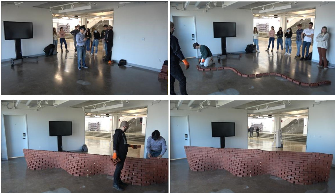
Figure 10 HoloMasonry wall construction
