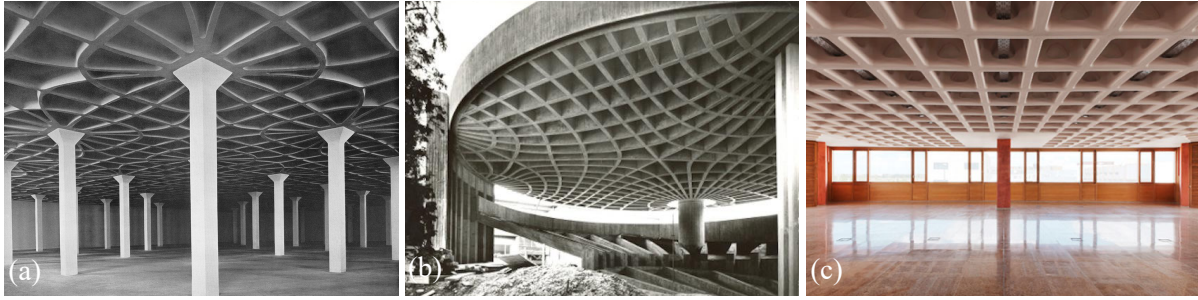
Figure 1. Ribbed building floors: (a) Pier Luigi Nervi's Gatti Wool Factory in Rome, Italy [1], (b) Hans-Dieter Hecker's Lecture Hall of the Zoology Department in Freiburg, Germany [2], and (c) Holedeck's modular waffle floor system [3].
