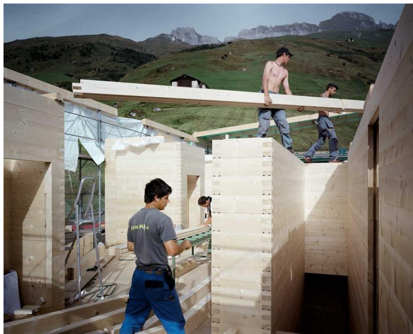
Figure 2: Manufactured by machine, assembled by hand: The Leis houses by Peter Zumthor are designed as a log construction. [© Walter Maier]
