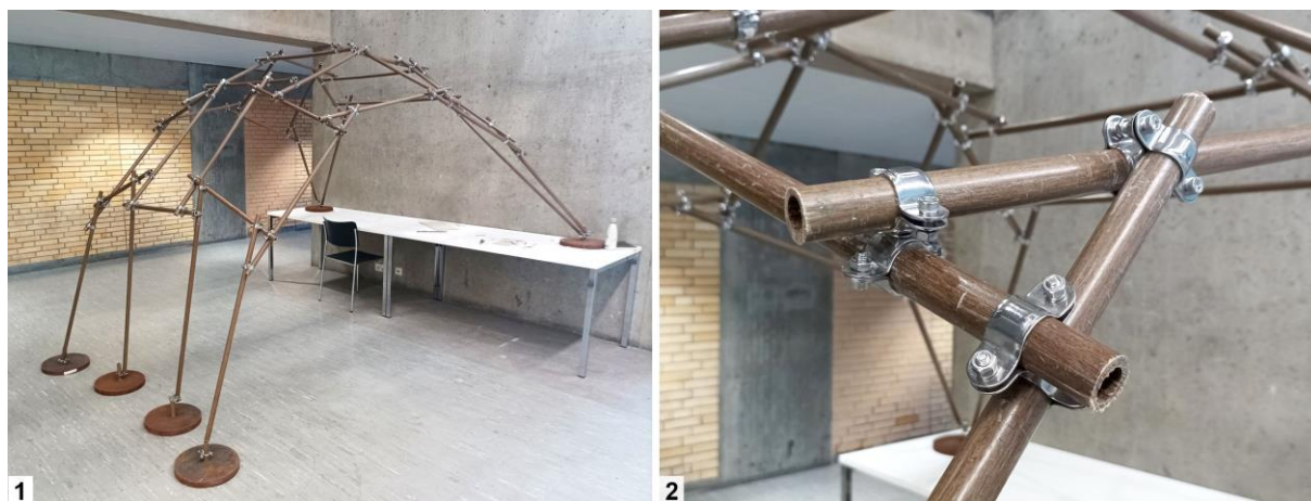
Figure 7: (1) Reciprocal Canopy Demonstrator 3x3x2 m, (2) three-member cluster joined with double-clamps
