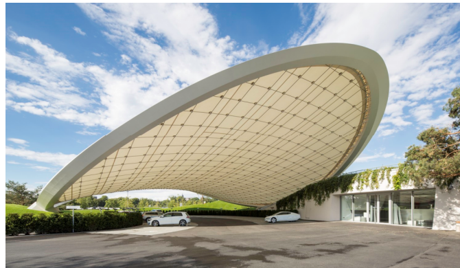
Figure 1: Autostadt Service Pavilion by Schlaich Bergermann Partner, © Tobias Hein, 2013
