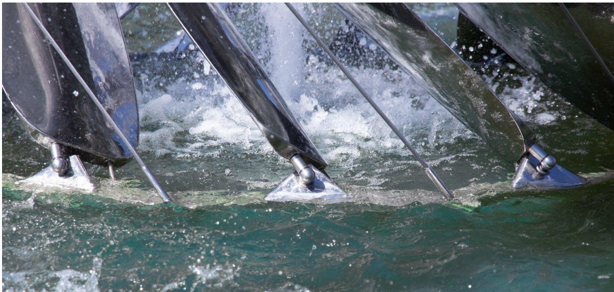
Figure 8: Lower node connecting the inflated steel elements and the ring beam [©Enrico Pontello].
