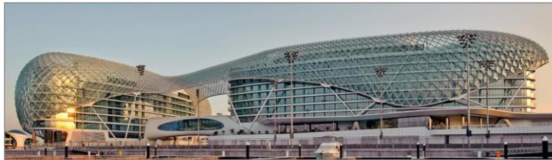
Figure 3: YAS Viceroy Hotel in Abu Dhabi (2008); structural design by schlaich bergemann and partner [2]
