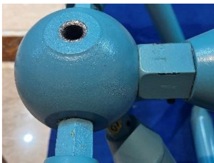
Figure 13: Traditional designed bolt-ball
