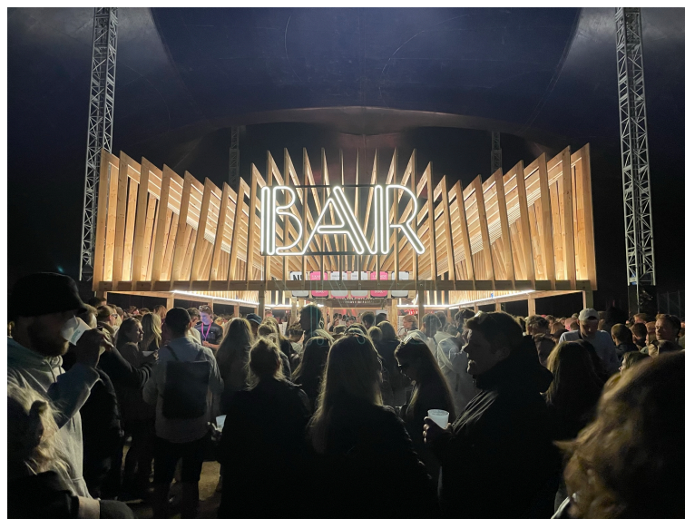
Figure 9: The prototype was designed with a roof construction made of pointy brackets to test warping and stability of the WasteBeams.
