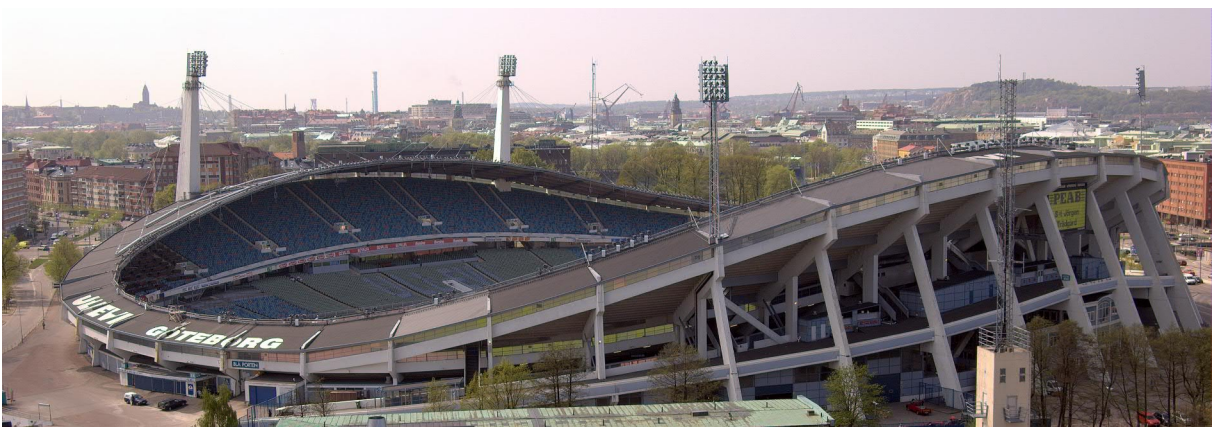
Figure 1: Ullevi as seen from the east with the pylons at the far end of the photo and the 1995 grandstand extension in the front. Photo [9].
