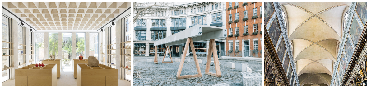
Figure 1: Abeille vault by AAU in Jerusalem © Mikaela Burstow ; post-stressed stone system by the Stone masonry company in London, retrieved from [1] ; groin vault in Santa Maria dei Carmini, Venice CC BY-SA 4.0 Didier Descouens
