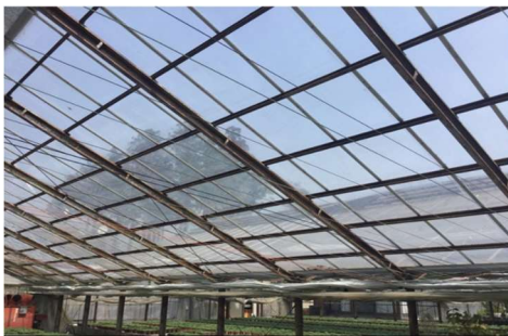
Figure 4 Photograph of a 60 \mu m ETFE greenhouse in use since 1988
