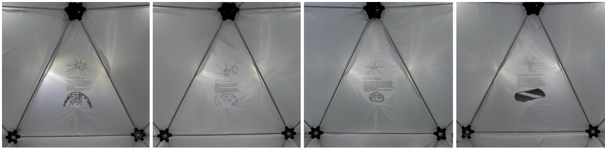
Figure 9: Textile prints of different space frame connector types on the inside of Puffer Dome
