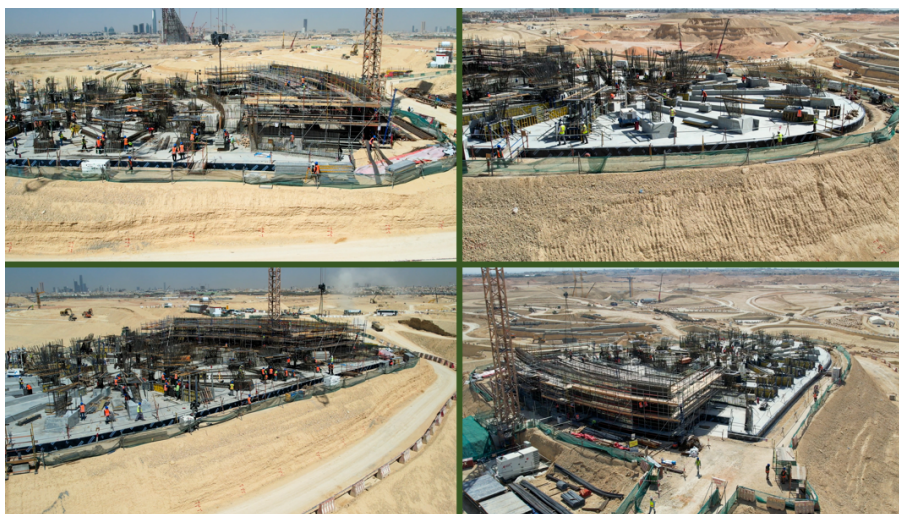
Figure 11: Construction progress at the Overlook site.
