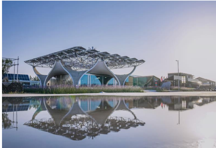
Figure 3: Photograph of Solar Ark 3.0
