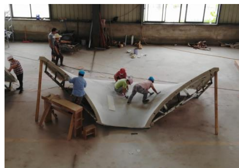
Figure 5: Fiberglass Formwork
