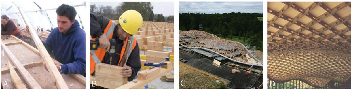
Figure 3 (A) Scarf-jointing the laths on site [16]. (B) Flat assembly of the grid on a scaffold and adding shear blocks [16]. (C) Lowering the scaffold and grid [17]. (D) Interior view of the finished Savill Gridshell [16].
