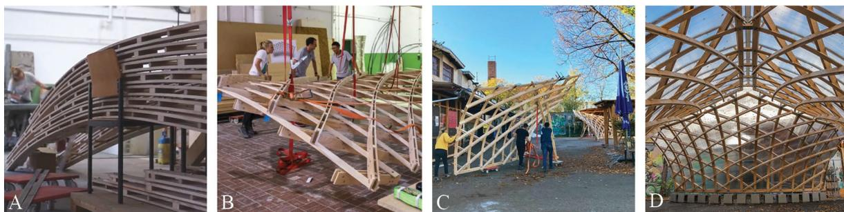
Figure 6: (A) Pre-bent asymptotic twin-lamellas. (B) Flat assembly and lifting/pushing the grid into the desired shape, the geodesic lamellas slide smoothly through the AA-Grid. (C) The modules were transported to the construction site and assembled with the other modules. (D) Interior view of the finished vault
