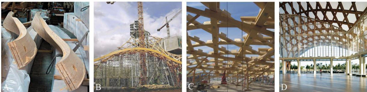
Figure 4: (A) Pre-bent, milled, double-curved beams [21]. (B) The entire construction process necessitated scaffolding for measurement and assembly [22]. (C) The prefabricated curved elements are gradually assembled on the construction site [18]. (D) Interior view of the Centre Pompidou Metz [21].
