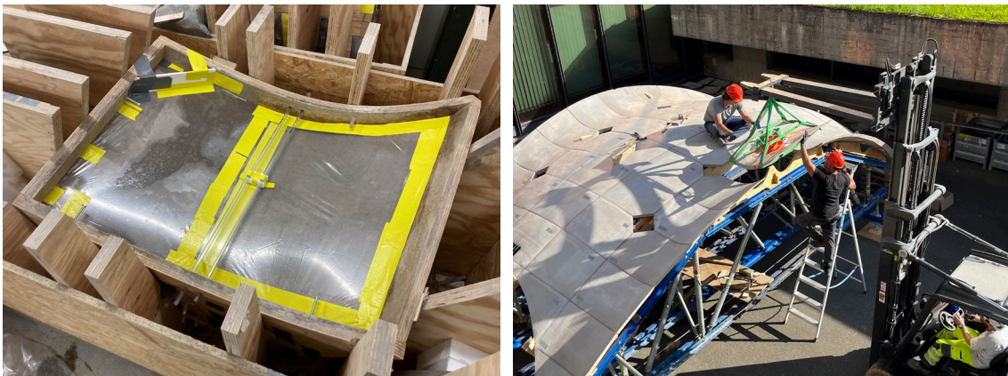
Figure 5: fabrication (left) and assembly (right) [©Lluís Enríque]
