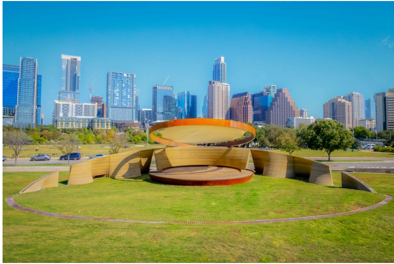
Figure 1: Performances taking place at the 3D-printed pavilion in Austin, TX
