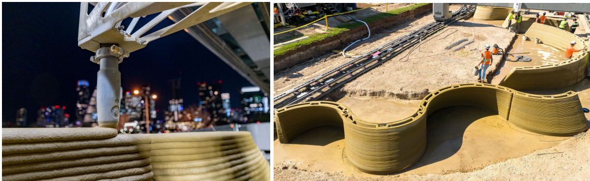
Figure 4: Construction printing an unsupported cantilever
