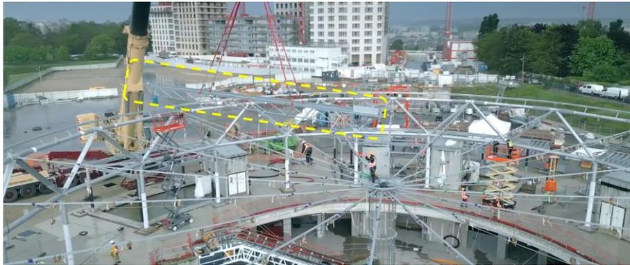
Figure 13: Installation of the polar maintenance beam, drone flight over construction site [credit: Bouygues]
