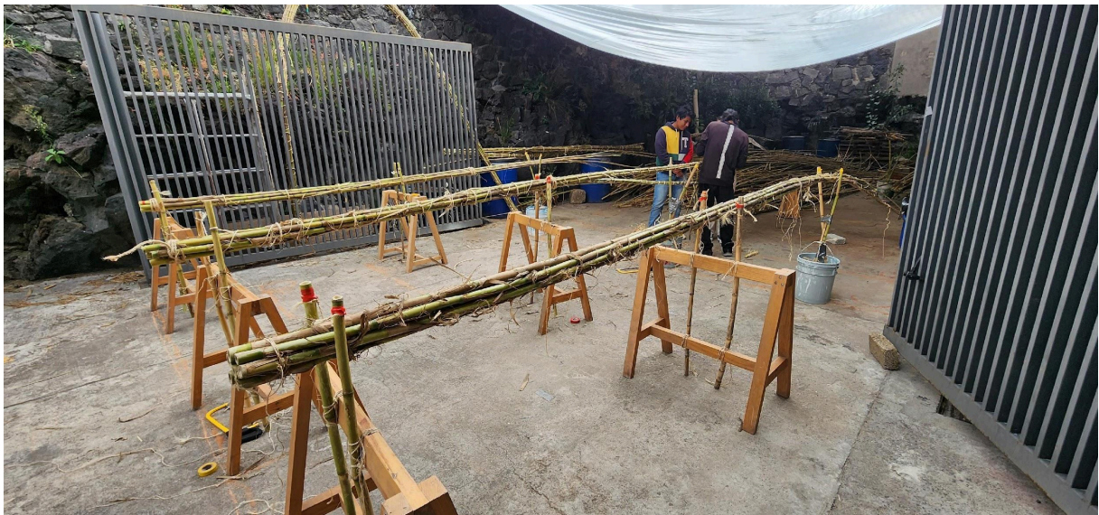
Figure 4: Assembly of reed modules [Photo: R. Bolaños]
