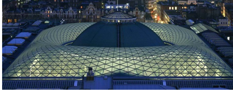
Figure 1: British Museum Roof, London, UK
