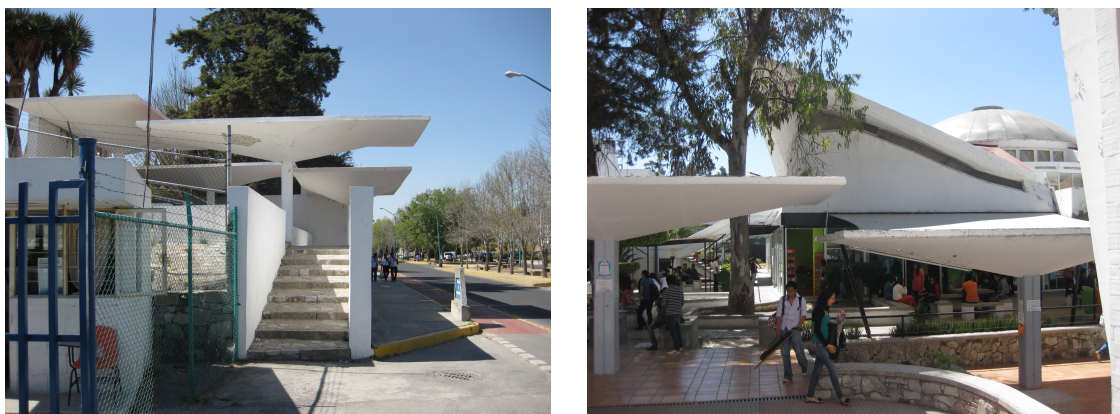
Figure 1 left: Umbrella-type hyperbolic paraboloids in the sports area of the BUAP university campus [2013]. Figure 2 right: Umbrella-type paraboloids and La Monja building at the Architecture Faculty of BUAP [2013].
