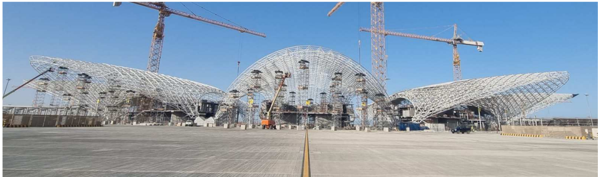
Figure 3: Space frame structure assembly completed
