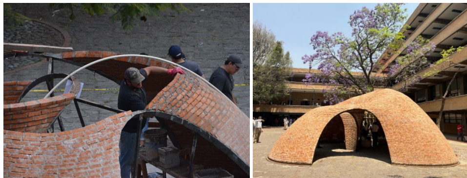
Figure 4: Constructing the experimental Pavilion PabUNAM and the finished brick vaults at the central yard of the Faculty of Architecture, UNAM.
