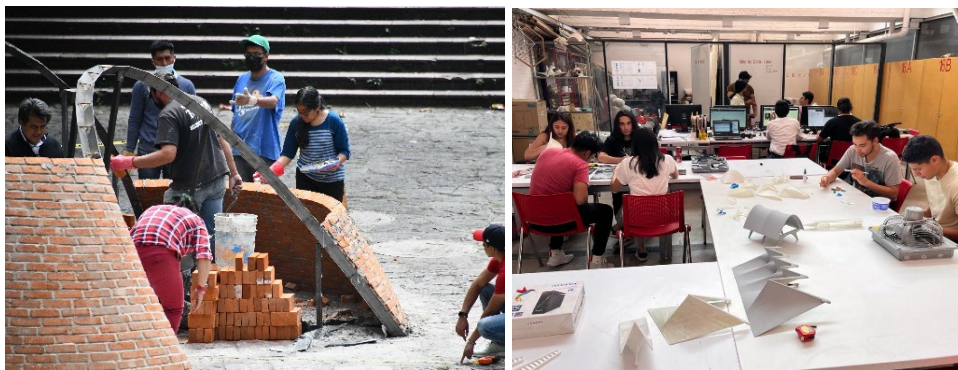
Figure 2: Students of the LSL Research Group working on constructing the experimental pavilion PabUNAM and preparing the exhibition of Candela's Legacy.
