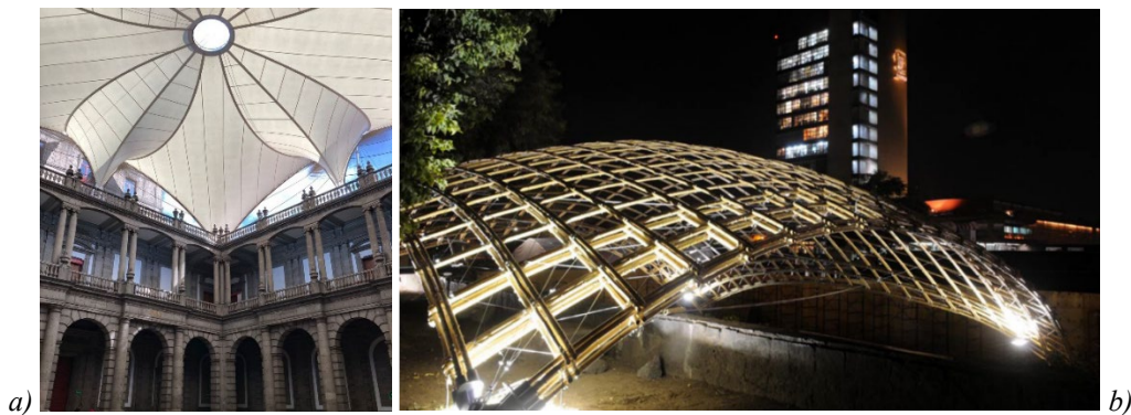
Figure 3: a) Tensile membrane structure for the central yard of the Palacio de Minería building. b) Bamboo gridshell at the UNAM Campus.
