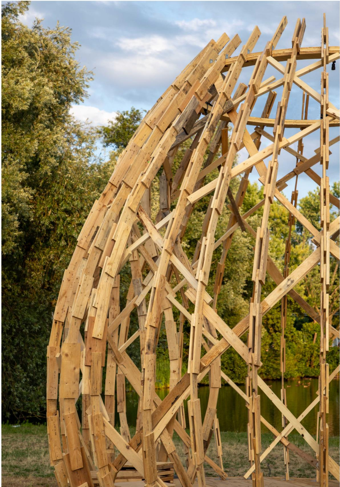
Figure 8: Nail-It pavillon for DasFest festival in Karlsruhe, structure
