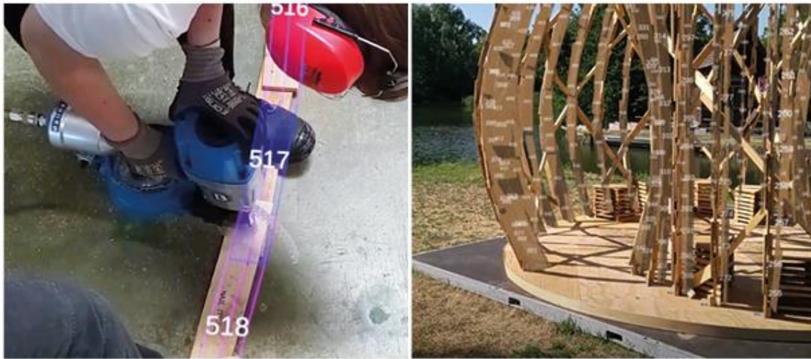
Figure 5: positioning and nailing of reclaimed elements according to digital template using AR (left) virtual and physical model of the final structure (right)
