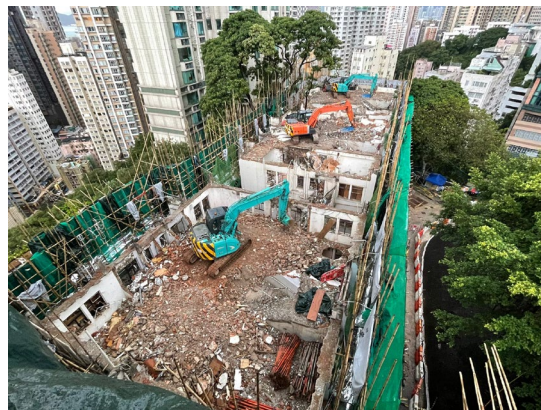
Figure 2. Demolition site photo
