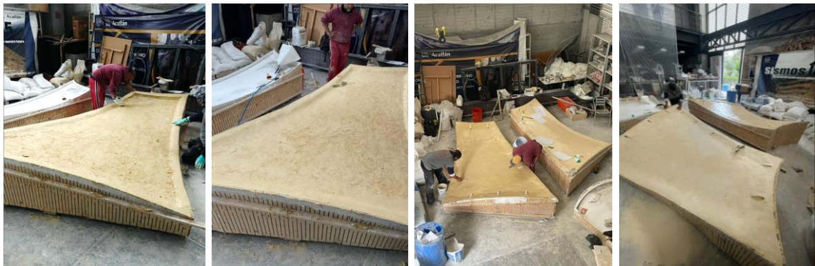
Figure 9: Segment casting process.
