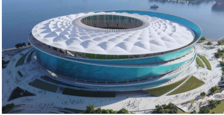
Figure 1: Photo of the gymnasium structure
