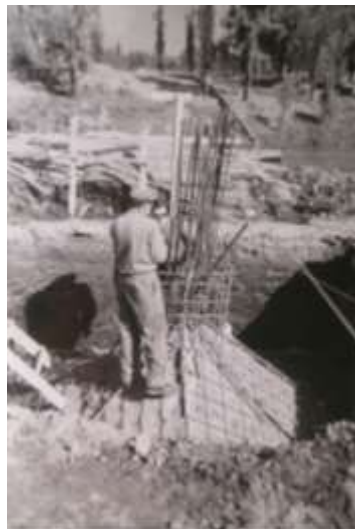
Figure 3. Los Manantiales shell umbrella footings.
