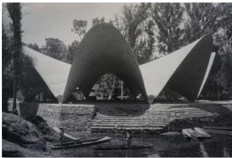
Figure 8: ‘Los Manantiales’ original masonry steps on the canal side.
