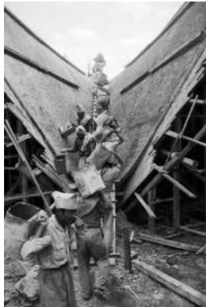
Figure 5. 'Los Manantiales' shell – concrete pouring by hand.
