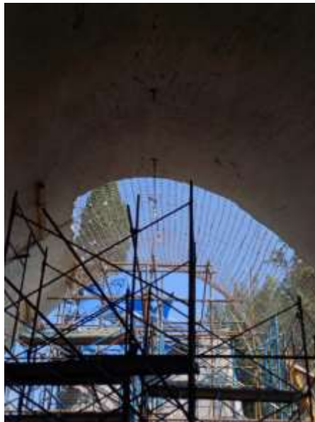
Figure 13: Partial demolition and repair of one of the ‘hypar’ shells.
