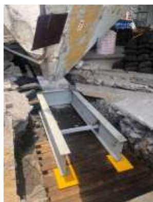
Figure 11: Existing footings connection with new radial tie-beams.
