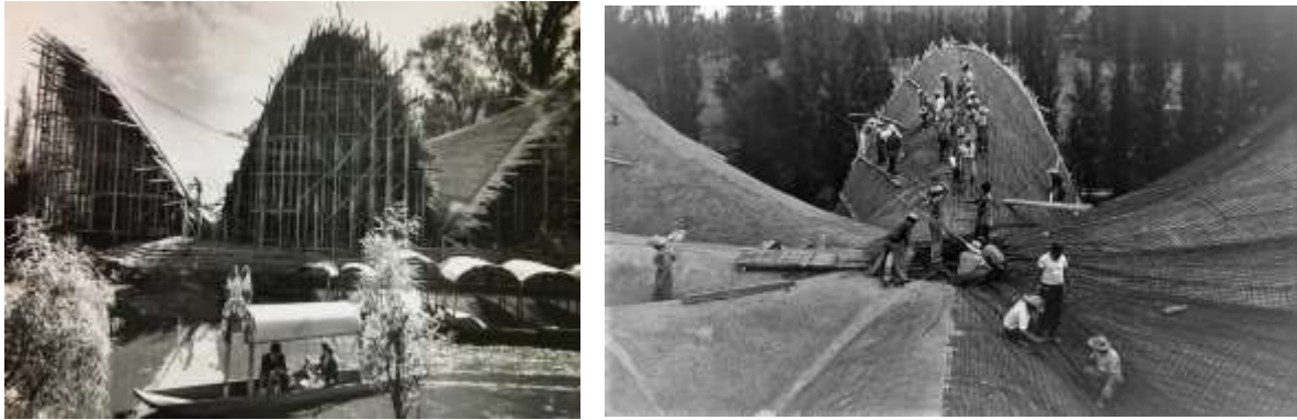
Figure 4. Los Manantiales formwork and shell steel reinforcement.
