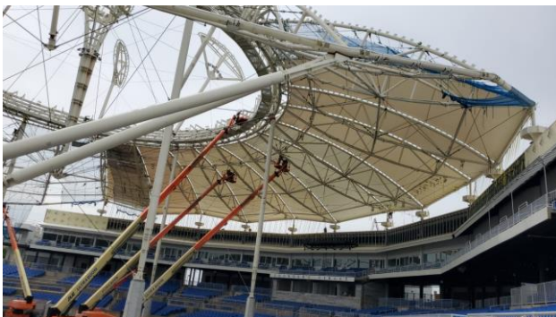
Picture 29 progress of skirt panels being installed. Picture 30 tensioning of skirt fabric panel.
