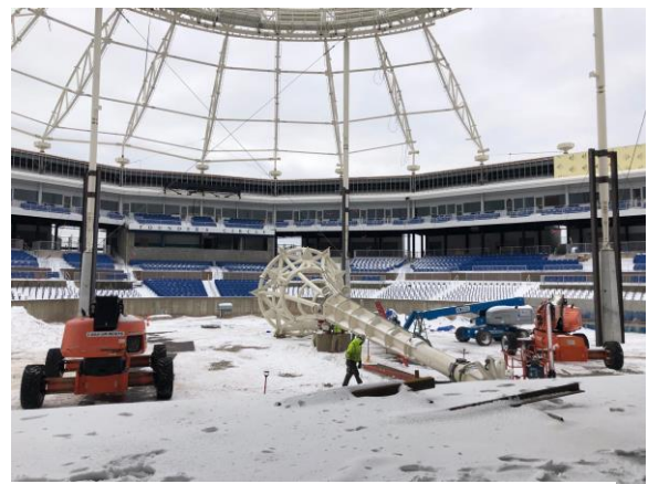
Picture 26 skirt erection and connection to ring. Picture 27 progress of skirt and main flying mast ready to lift.
