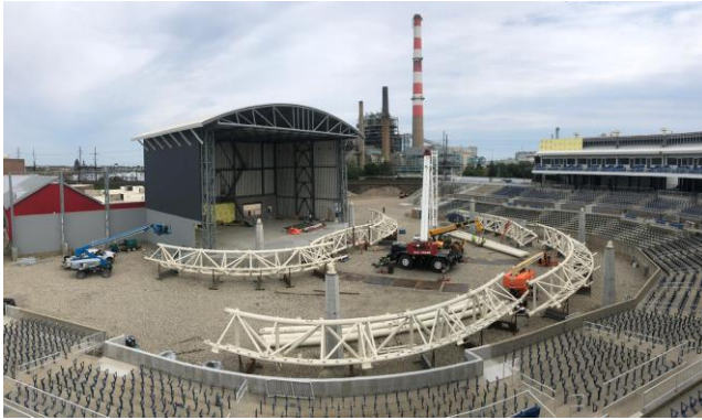
Picture 25 unload sections of ring ready for erection. Picture 26 last section of ring been install.
