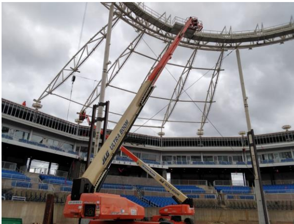
Picture 26 skirt erection and connection to ring. Picture 27 progress of skirt and main flying mast ready to lift.
