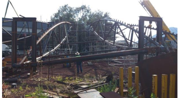
Picture 19 Pre-assembly of ring before ship to site. Picture 20 Pre-assembly of skirt before ship to site.
