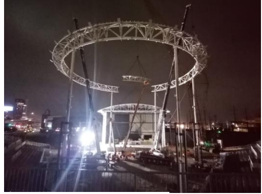
Picture 25 unload sections of ring ready for erection. Picture 26 last section of ring been install.
