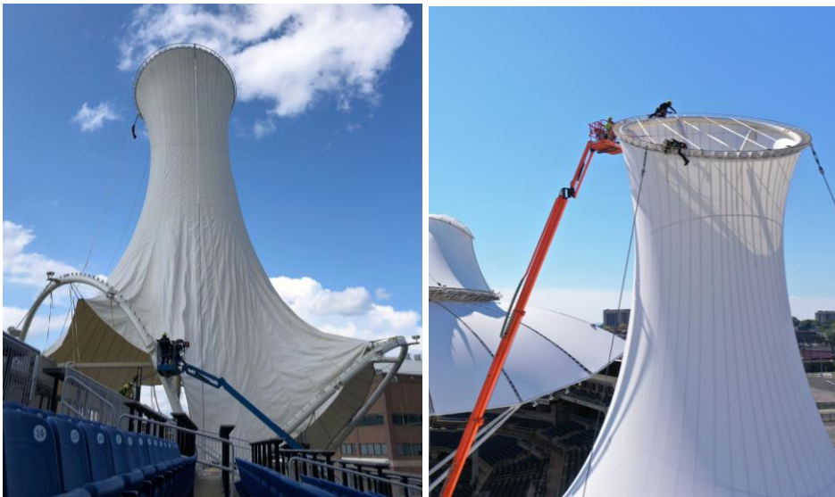
Picture 33 process of the entrance pavilion been tensioned. Picture 33 preparation for the ETFE skylight to be installed.
