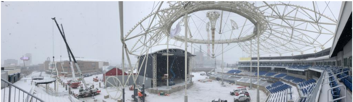
Picture 28 The completed main steel structure along with the flying mast, which awaits the arrival of summer for fabric installation. Additionally, cranes working diligently to erect the entrance pavilion.
