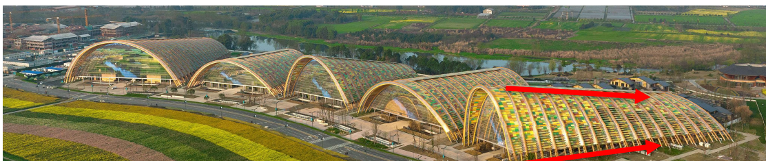
Figure 9: Sloped ridge lines added complexity
