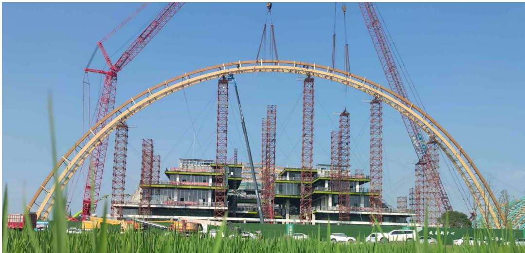
Figure 16: G1, second arch (115m)
