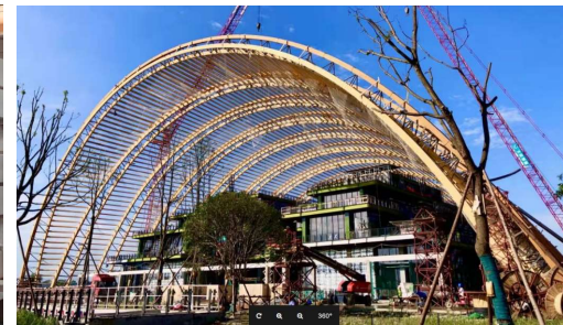
Figure 11: Smooth enclosure, optimized purlin distribution
