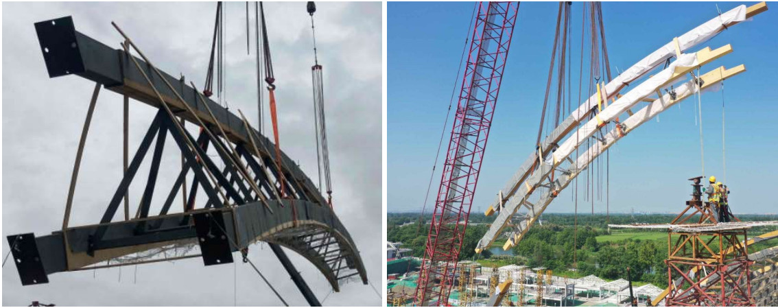
Figure 15: Lift-assembly and shoring tower
