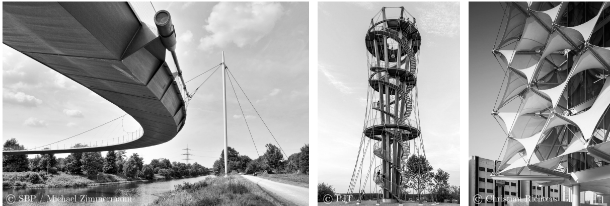
Figure 1: Lightweight structures are assemblies of distinct substructures and typologies. Left: a cable-stayed bridge. Middle: a post-tensioned observation tower. Right: a membrane shading system.
