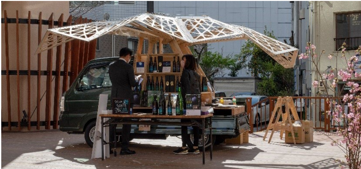
Figure 5: Deployable roof for a food truck (osake-mushi). (S. Shibata, S. Nakamoto, K. Saito, Suzusan Zaimoku, VUILD, 2022)
