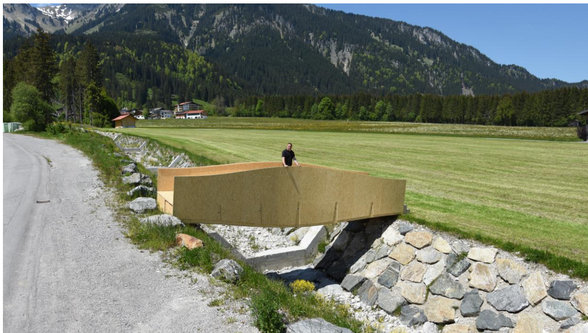
Figure 12: The final bridge spanning over a small river
