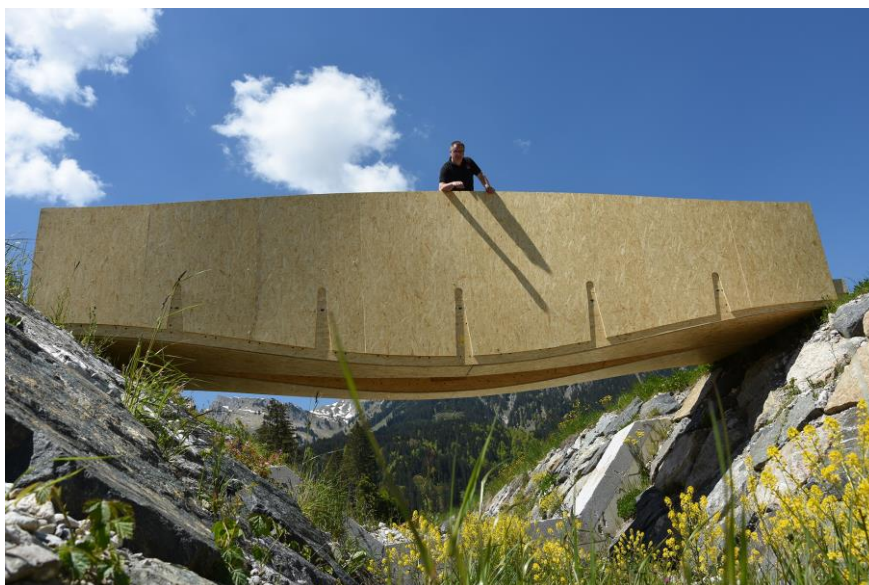
Figure 1: the bridge on site
