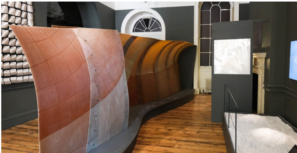
Figure 2: ‘Creative Differences’ pavilion in LDB2023 featuring ‘The Swirl’, a frustrated composite partition.
