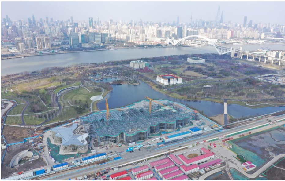
Figure 22: Construction Photo ©Yiju Ding
