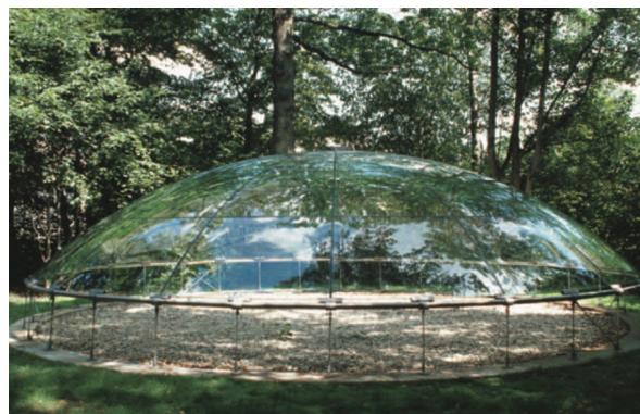
Figure 3: The glass panes are actively involved in load transfer in this Stuttgart glass shell. [10].
