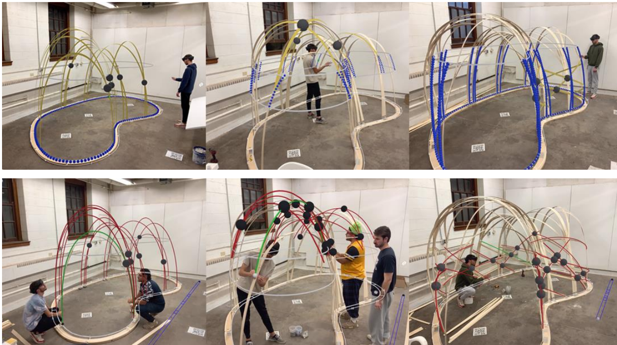
Figure 6: Sequential assembly with mixed reality guides developed in real time. The team switches from design mode (top) and fabrication mode (bottom).
