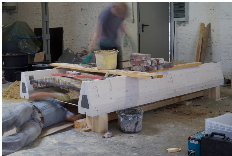
Figure 3: 1:1 Demonstrator of a transformed Prussian capped ceiling between specially milled timber beams at ZukunftBau Pop-up-Campus Aachen, 2022.
