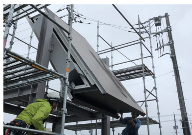
Figure 24: Façade mock-up
