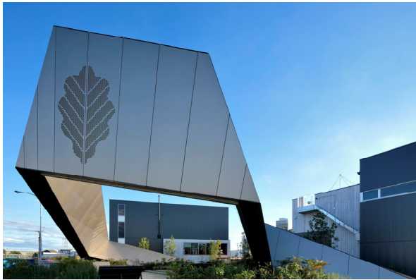
Figure 3: View from the west
