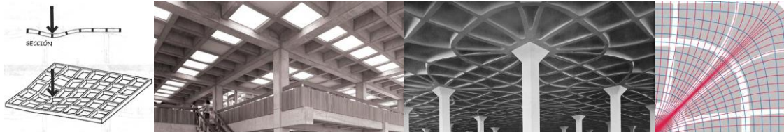
Figure 2: From left to right: sketch showing orthogonal ribs causing torsion to each other (Moore [5]); comparison between slabs with thick, orthogonal ribs (PUCMM Library in Dom. Rep., built by F. Camarena in 1975 [11]), and slabs with thin, stress-aligned ribs (Gatti Wool Factory in Italy, built by P. L. Nervi in 1953 [12]); and diagram showing how the ribs of the latter are aligned to the principal stress lines (Halpern et al. [13]).
