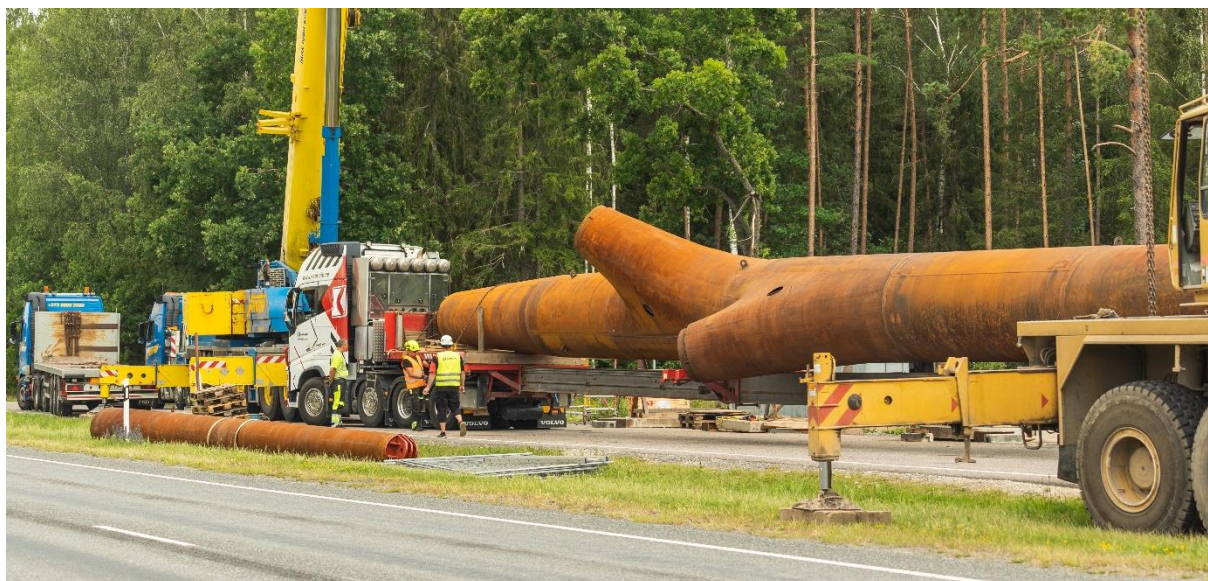
Figure 4: Transportation of individual pylon segments [Image: ©Estfilm, Lauri Nagel]
