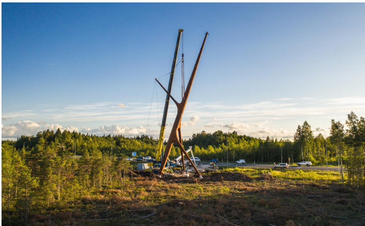
Figure 3: Assembly and erection process during construction [Image: Estfilm, Lauri Nagel]
