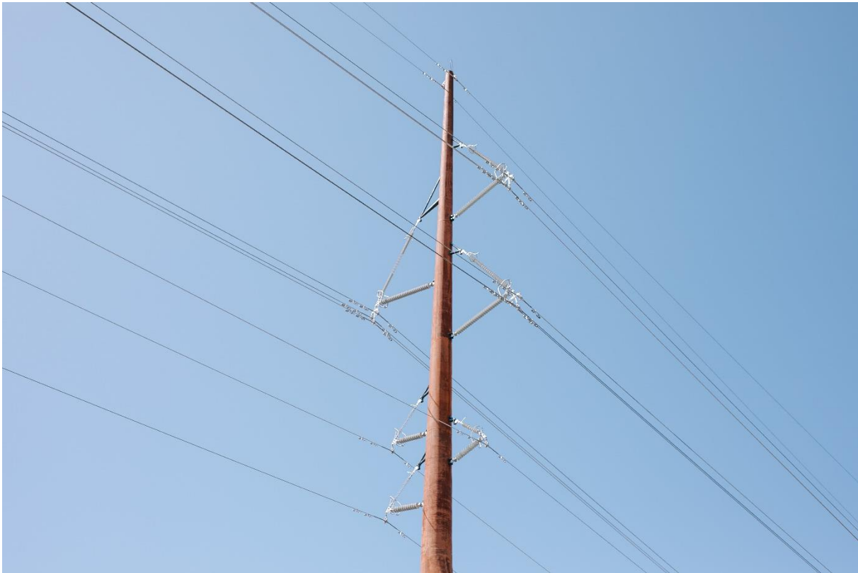
Figure 6: Attachment details of electric isolators and V-shaped mounting points [Image: PART Architects]
