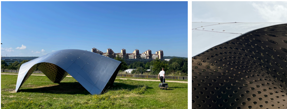
Figure 1: Air Foil Pavilion - Demonstrator made out of two layers of 0.8mm stainless steel sheets
