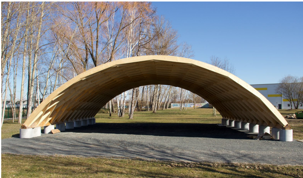
Figure 1: Demonstrator based on the ReFlexRoof principle (TimberPlan+) [FLEX @ HTWK Leipzig, M. Zwigart]
