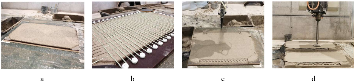
Figure 5: a) First cover layer SC3DP, b) Fiber reinforcement frame placement, c) SC3DP of effective concrete mass, d) Green-state surface smoothing by CNC-troweling
