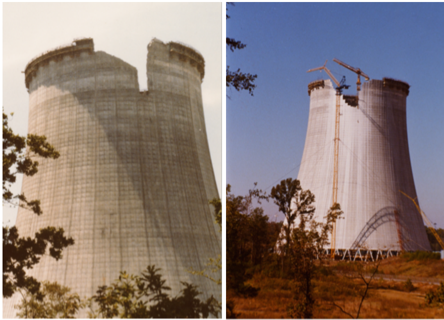
Figure 1: The damaged cooling tower and the restored crane during repair [1].
