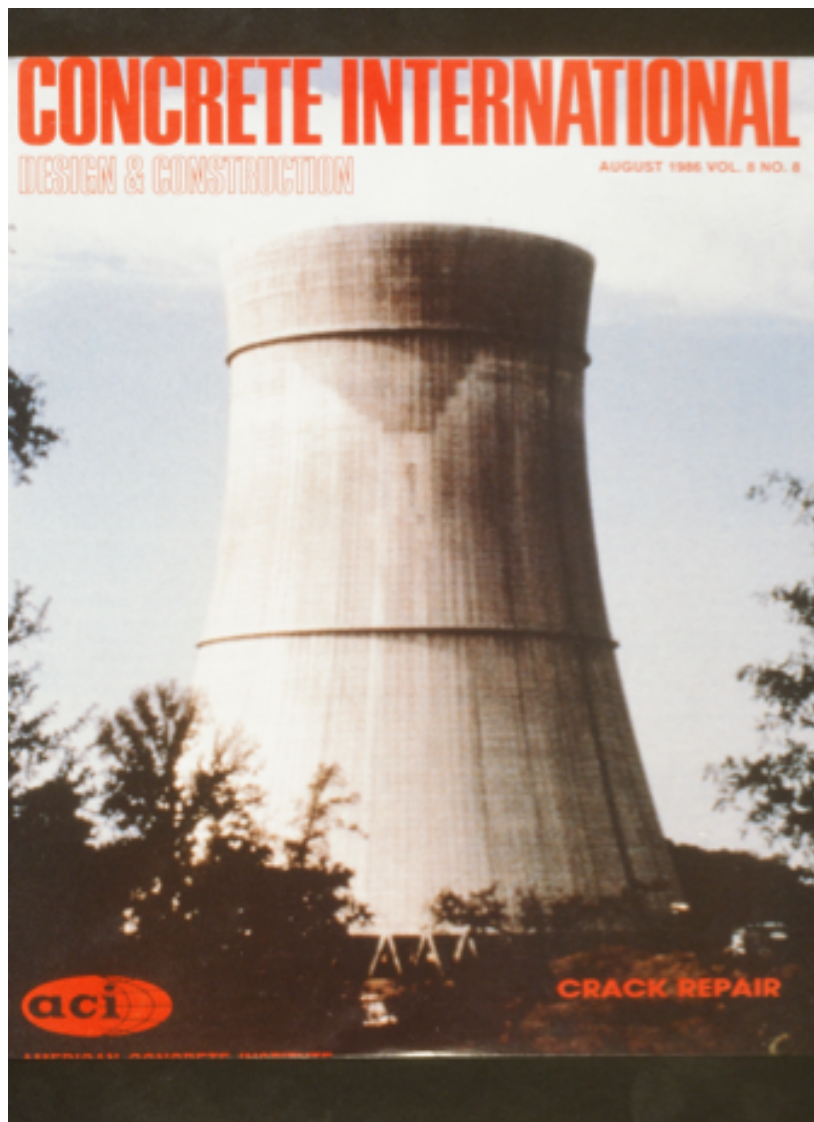
Figure 4: Completed Structure.[Concrete International,ACI]
