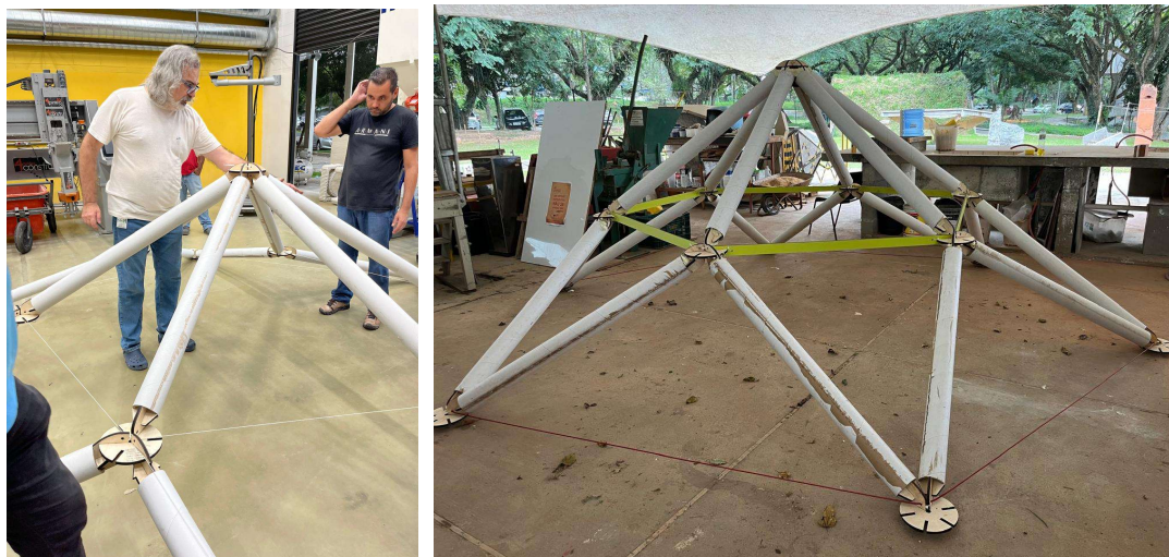
Figure 14: Reticulated polar zonohedron under construction
