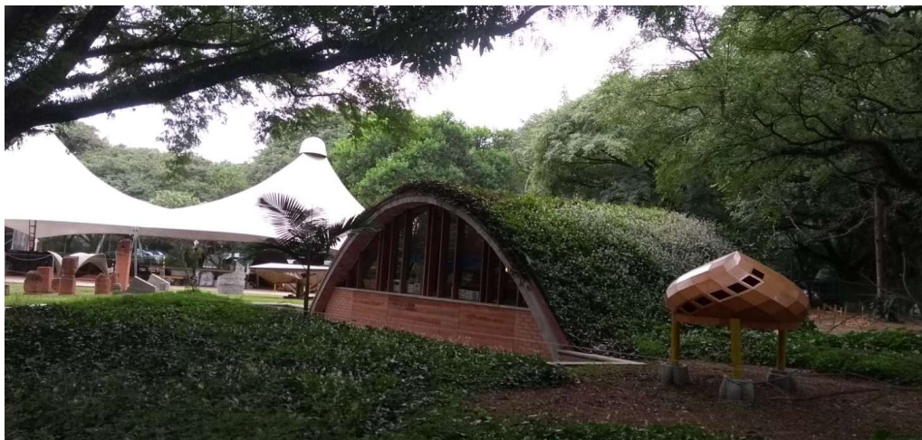
Figure 12: Continuous polar zonohedron composing the landscape of the Laboratory of Constructive Culture
