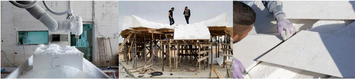
Figure 22: (left) polystyrene blocks carved. (center) timber formwork and polystyrene blocks. (right) placing of stone voussoirs
