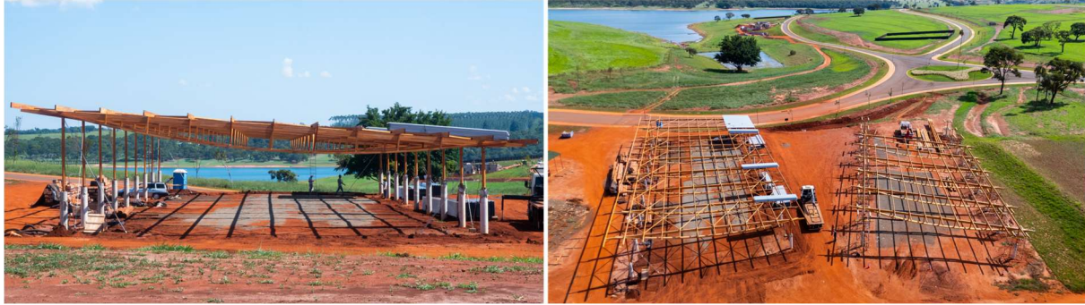
Figure 20: Finishing assembly and starting roofing process.
