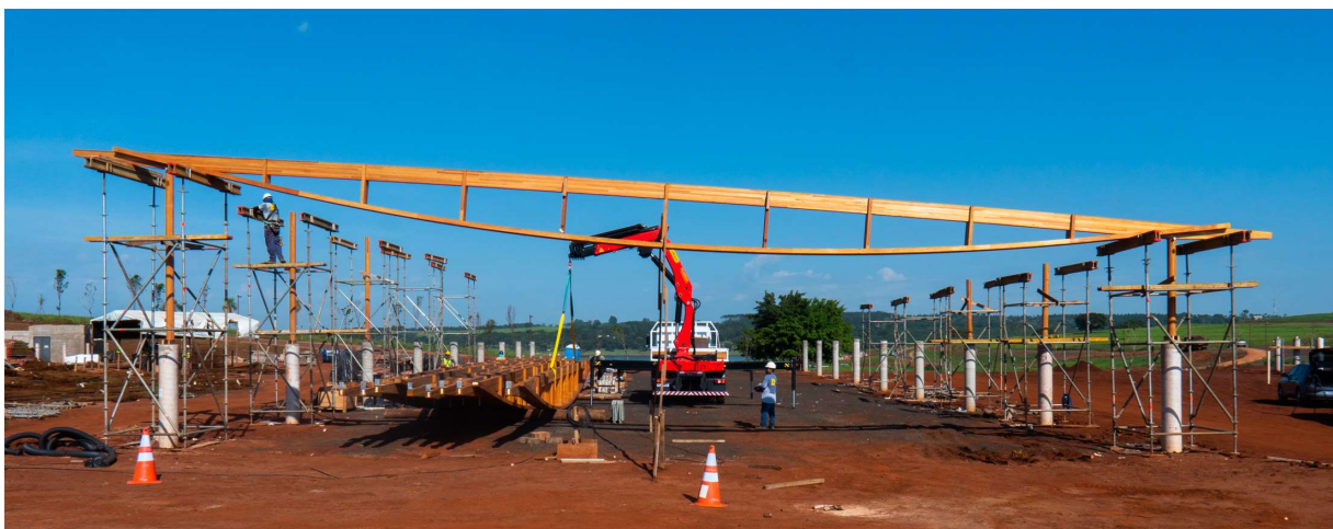
Figure 1: first beam-string assembled on site.
