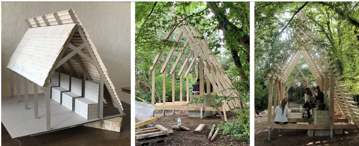
Figure 9. Final pavilion design and build: physical model and framing in progress.
